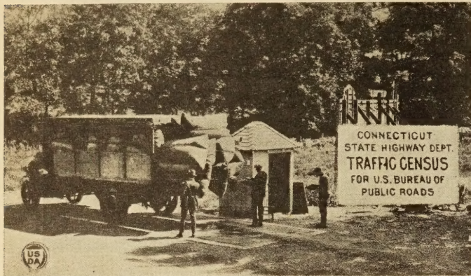
An intensive weighing station. Observers weighing and measuring a 4-ton load of rabbit fur, bound from New York City to Norwalk, Conn., 44 miles.
